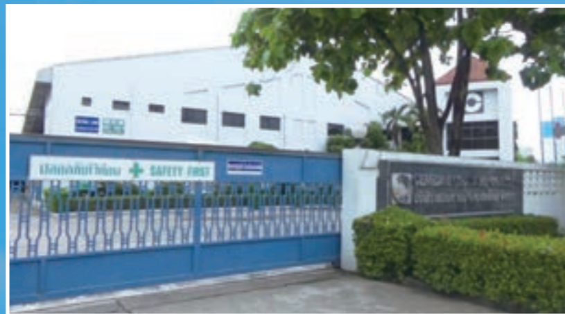
Establishment of Cemedine (Thailand)
