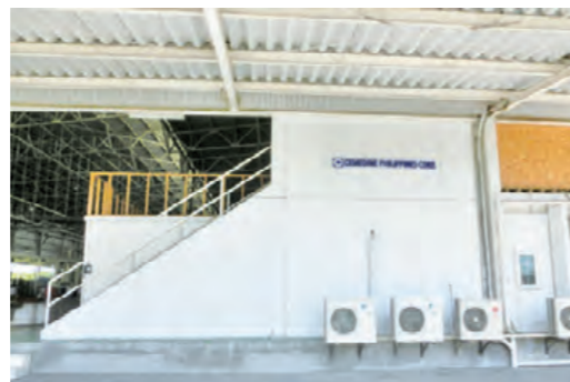
CEMEDINE PHILIPPINES CORP. Block2, Cavite Eco-ZoneII, General Trias, Cavite, Philippines 4107
